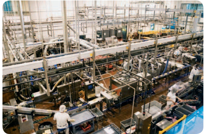
Stainless steel chains used in a cheese processing plant
