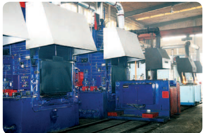
Furnaces for heat treatment process
